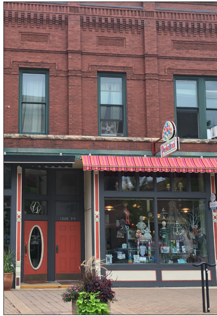
Cast iron SHOPFRONT with brick second STORY
