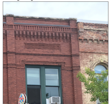
Parapet walls with projecting brick corbels
