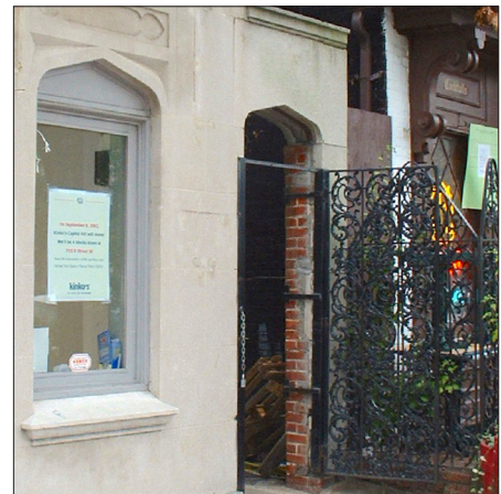
STREET WALL with gate
