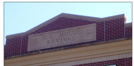
Masonry parapet sign
