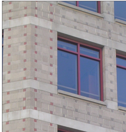
Windows recessed behind FACADE surface
